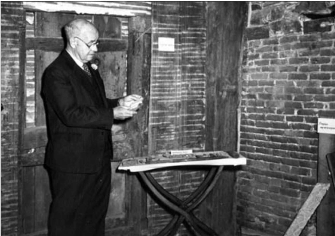
John Hutchins Cady in the Richard Smith Jr. Room, 1951. A Providence architect, Cady led the first renovation of the Castle by the Association in the 1950s. To the right are fragments of 17th century paneling (marked "Original Sheathing") that Cady replicated on all the walls in this room. On the table are artifacts discovered behind the plaster lathe. Behind him is a blocked-up doorway that remains hidden under paneling today. This is one of several photos from the 1950s restoration in the Castle archives.
