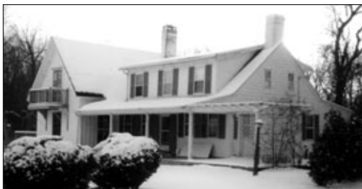
The house in which the Pitmans lived at Duck Cove remains, albeit in an enlarged and modernized condition. Photo courtesy of Natalie Richmond Hamlin.
