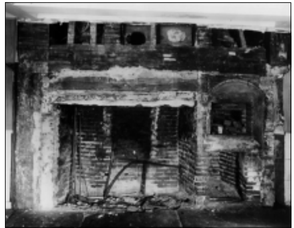
Figure 2. The Isham drawing appears on the reverse of this photo with the note: "Cocumscussoc. Nov. 1, 1926 / Photo taken by Anty./ Kitchen fireplace after Mr. Fox had taken out one fireplace, traces of which are seen as the back of the present (Nov. 1) fireplace. / N.M.I." Photo courtesy of the Rhode Island Historical Society (RHI(x3)2997).
