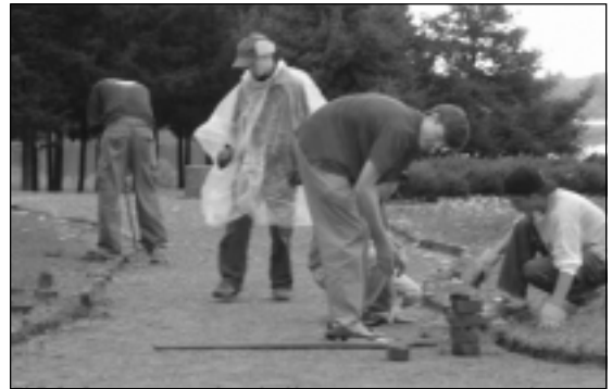
Castle Walkways receive a much needed upgrade by members of Scout Troop 152. Their work was coordinated by Gregory Nannig, second from right.
