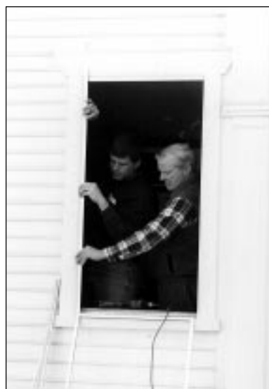
Dick Bowen helps Tom Haling of New England Glass and Mirror install new storms and screens on Castle windows. Photo by Barbara Carey.
